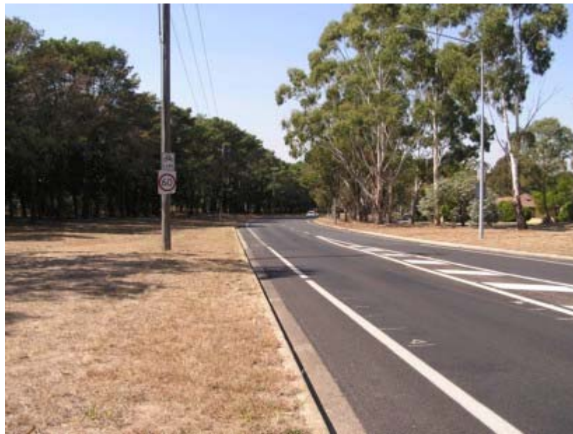
Owen Dixon Drive, Evatt, showing new cycle lanes marked during routine resealing
